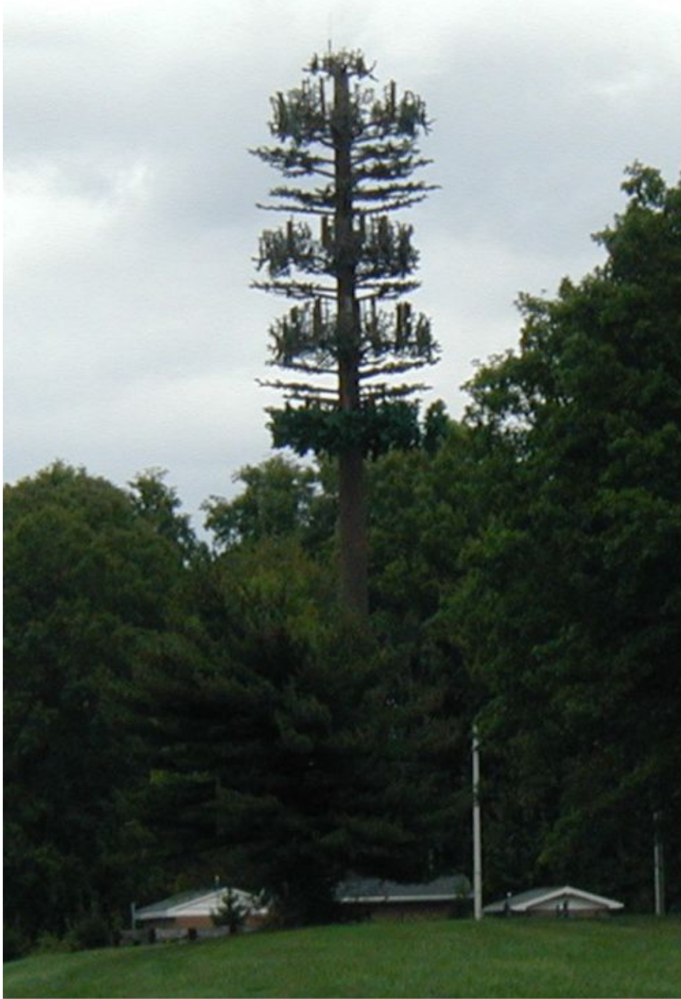
Figure 8.3: Cell phone tower disguised as a tree.
